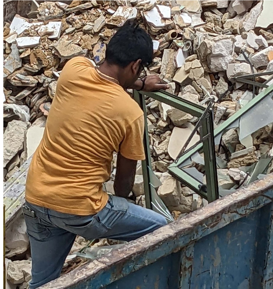
Figure 7: Worker Removing Glass with Bare Hands
